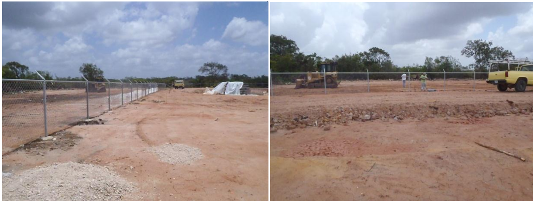
Perimeter chainlink fence progress
