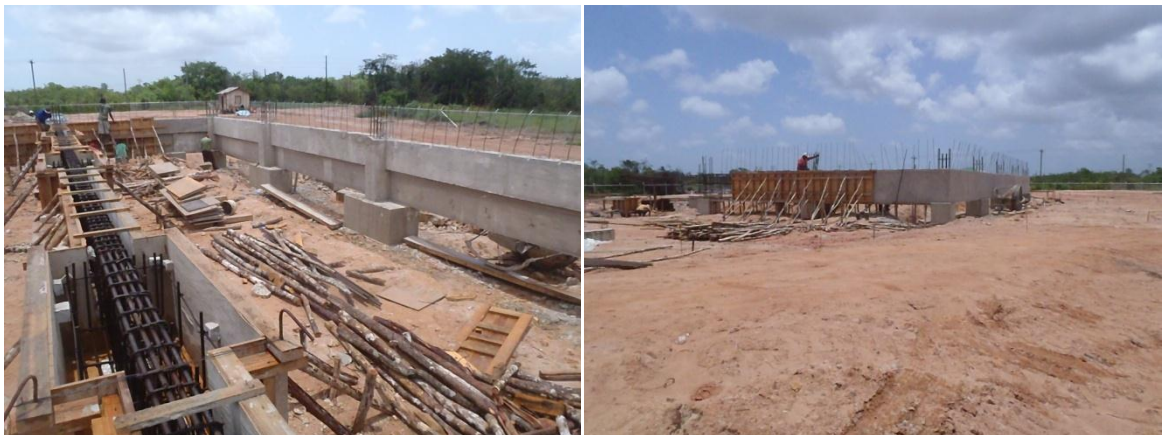
Transfer Station progress of in-situ concrete beams
