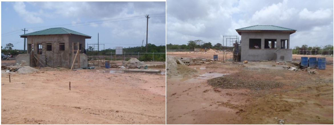
Administration Building Construction Progress
