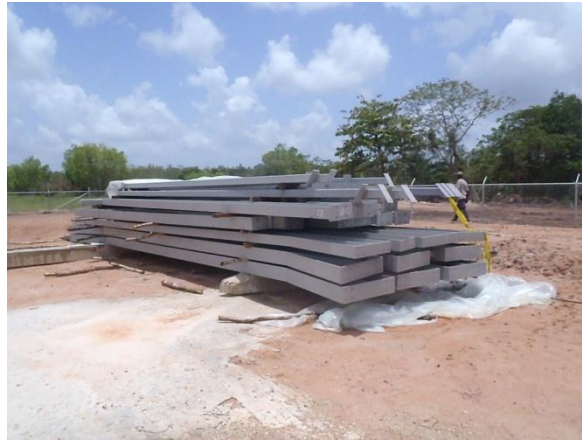
Transfer Station steel frame members on site.
